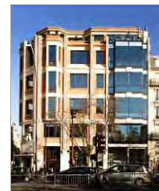
InPost 5 100 m 2 HON Hines France / Carrefour Property
